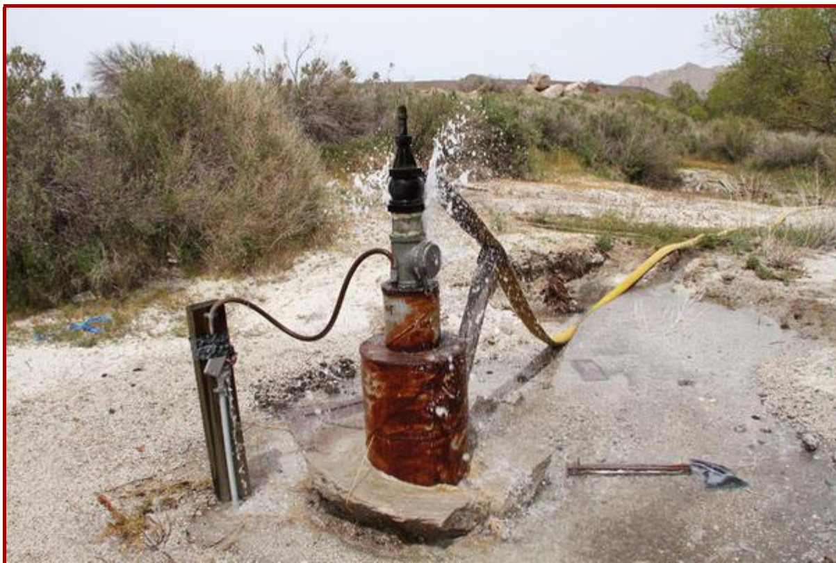
Fig. 25 Jacumba Water District's well head, flowing under artesian conditions on April 17, 2010.
