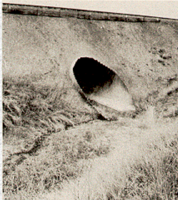
Figure VI-33--Unanchored Mitered End
