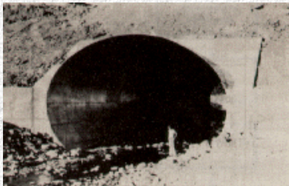
Figure I-2--Long Span Culvert
