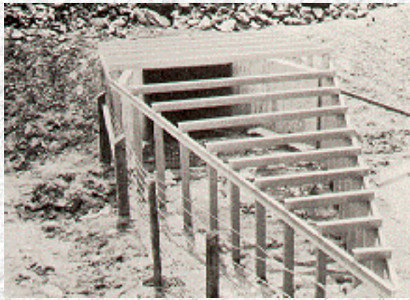
Figure VI-16--Debris Deflector
