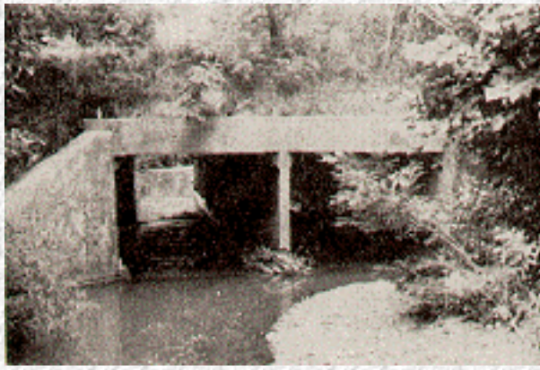
Figure VI-21--Double Barrel Box Culvert
