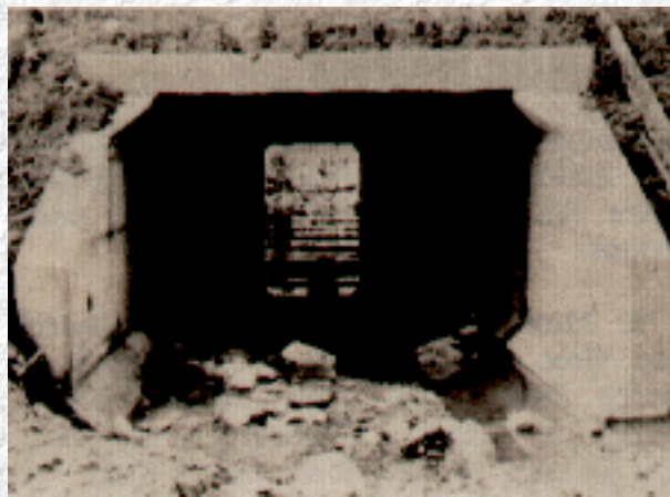
Figure I-5--Precast Concrete Box Culvert (American Concrete Pipe Association)
