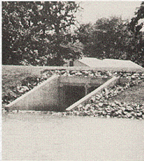
Figure VI-1--Stormwater Management Pond with Culvert as Outflow Control Device
