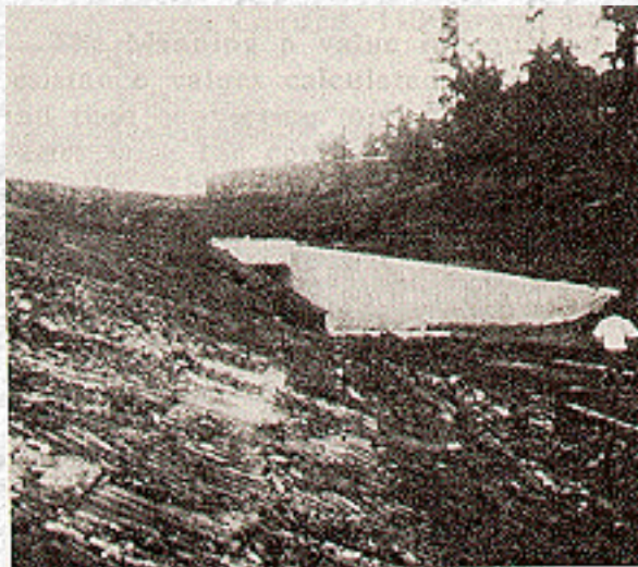
Figure VI-20--Fill Warped to Avoid Inlet Skew
