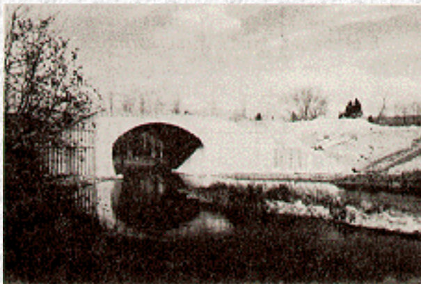
Figure VI-10--Culvert with Metal Headwall and Wingwalls (ARMCO)
