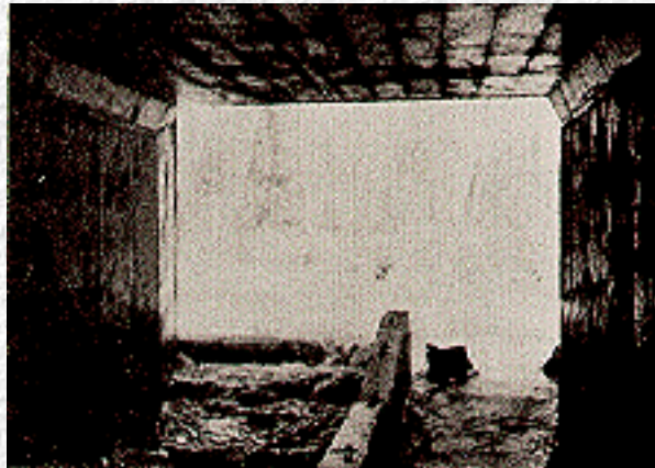
Figure VI-7--Fish Baffles in Culvert
