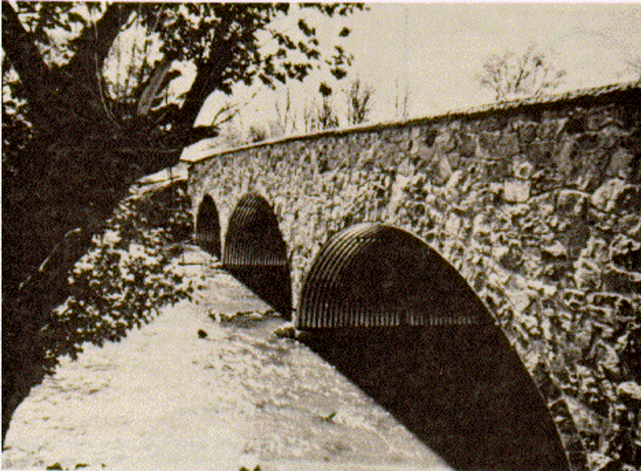
Figure I-6--Corrugated Metal Arch Culvert (ARMCO)
