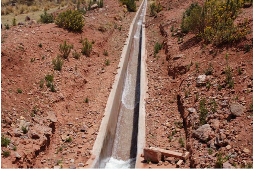
Fig. 5 Roll waves traveling in a steep irrigation canal, Cabana-Mañazo, Puno, Peru.
