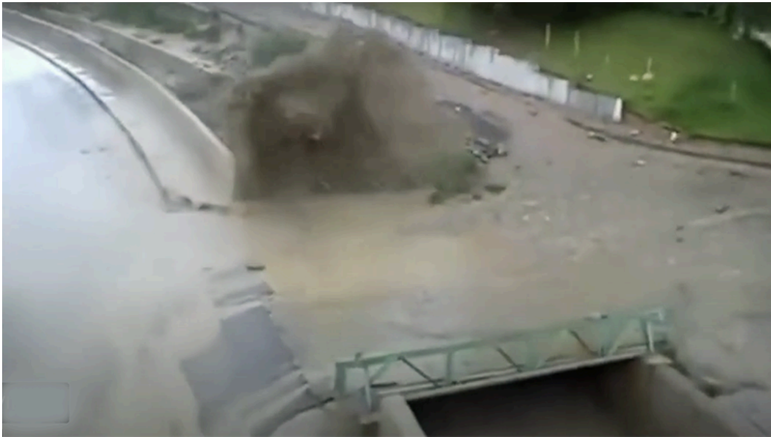
Fig. 6 Roll waves, also referred to as pulsating waves, overtopping the Huayñajahuira river channel, in La Paz, Bolivia, on December 11, 2021.
